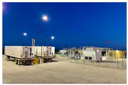
Operations utilizing a centralized RNG collection station. An enclosed compressor ads the renewable natural gas into tube trailers for transport to a site or a J-W Power company compressor to inject into the pipeline.
